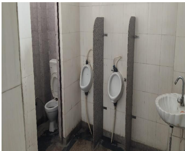
3 rd Floor Boy's Washroom
